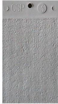
CSP-3: Light Shot Blast/ Bush-hammering
