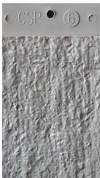
CSP-6: Medium Scarification
