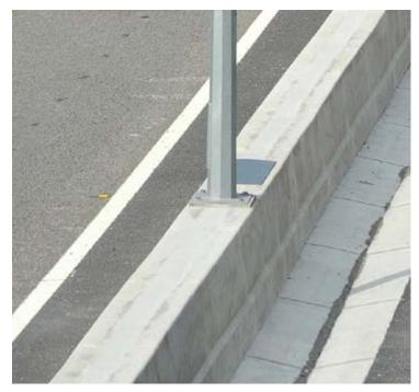
Sika concrete admixtures are playing an important role in the upgrading of central crash barriers on the UK's motorway system. Since 2005, the Highways Agency policy has been that high-containment concrete step barriers be used for all central reserves on new motorways and as replacements for barriers that have reached the end of their useful life on existing motorways.
