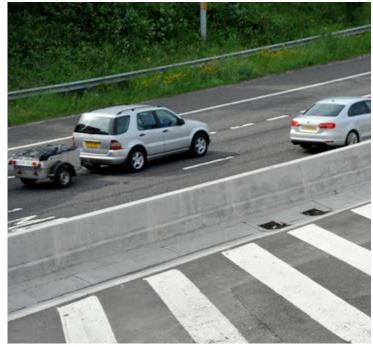
To help with any future freeze/thaw issues associated with the aggressive motorway environment, a Sika air entraining admixture was also added to the mix. This adds air within the structure and reduces the internal stresses caused when the structure is exposed to freezing conditions and thus preventing any damage from the freeze/thaw cycle.
