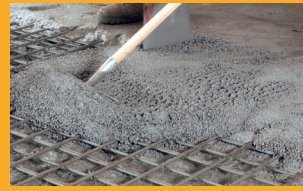
CONCRETE AND REPAIR
