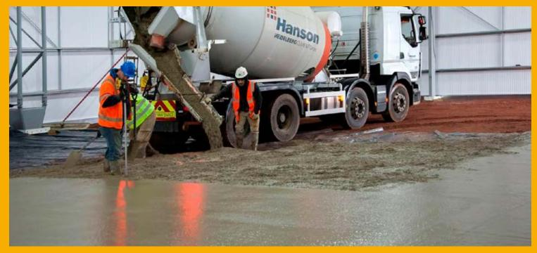
Working with contractor NEM Plant, Sika and Hanson recommended the use of both the Sika<sup>®</sup> VisoCrete<sup>®</sup> admixture to provide good workability and Sika<sup>®</sup> Durus Macro Fibres, as an alternative to steel mesh, as the space on site was limited and the timeframe was crucial.
