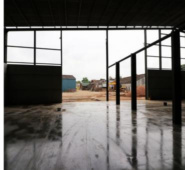
The concrete was placed using laser guided screed machinery and power-floated to achieve a buffed and polished finish, before contractors applied Sikafloor<sup>®</sup> Proseal curing agent to enhance surface finish and hardness.
