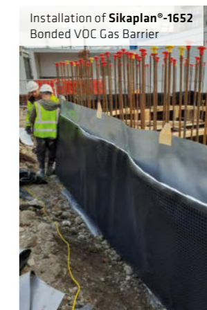
Installation of Sikaplan®-1653 Adhered VOC Gas Barrier
