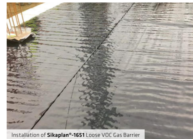
Installation of Sikaplan®-1651 Loose VOC Gas Barrier
