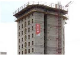
**Improved Early Strength for Slipformed Concrete** Speeds up the construction process
