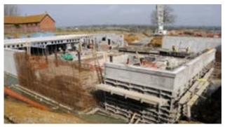
**Early Strength for Increased Formwork Rotation**Reduced cost and shortened stripping times
