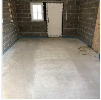
One of the key benefits of RMX Ezi-Flo is its ability to be placed directly from the delivery wagon chute, finished with a dapple bar and sealed with curing agent; a rapid alternative to the timely and costly traditional method of physically placing the material, levelling with machinery and allowing for the requisite curing time.
