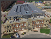
SINGLE PLY ROOFING
