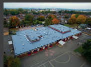
LIQUID APPLIED ROOFING
