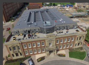
SINGLE PLY ROOFING
