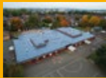
LIQUID APPLIED ROOFING
