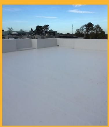
mechanically-fastened membrane was affixed to the building's decking using Sika-Trocal's unique laminated metal discs. The waterproofing system was augmented by Sika-Trocal INNOfix, a high performance, foil-faced tapered insulation. Sika's S-Vap 500E provided the non-decaying, unsupported, vapour control layer.
