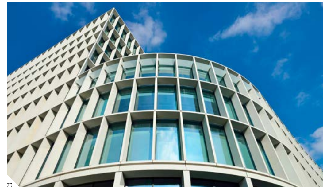
One New Ludgate Project participants Architect: Fletcher Priest Architects Facade: Josef Gartner (2016)
