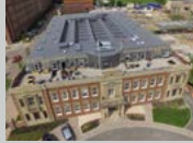
SINGLE PLY ROOFING
