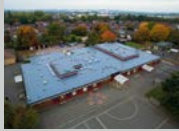
LIQUID APPLIED ROOFING
