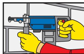
1. Drill hole with an electric drill to the diameter and depth required. Drill hole diameter must be in accordance with anchor size.
