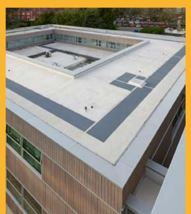
Sika-Trocal's vapour permeable membrane was mechanically fastened at the perimeters and around penetrations using the product's innovative laminated metal disc system. This system sees the membrane fixed to the roof in a single process, ensuring a fast installation, minimising components required and reducing overall project costs. A 120mm thick, high performance rigid thermoset insulation was also applied to improve the thermal efficiency of the buildings.
