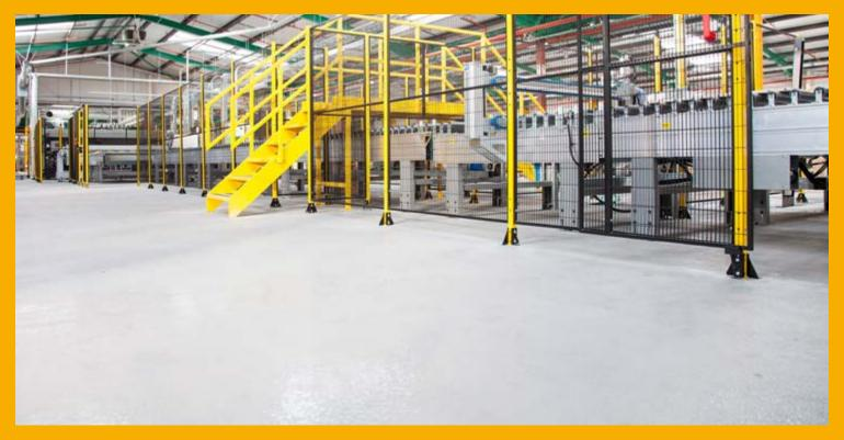
Main contractors, Zircon Flooring, specified Sikafloor®-264, a two-part epoxy roller and seal coloured-coat, which comes with a guarantee and provides the ideal hard-wearing surface for concrete and cement screeds. Its anti-slip properties were particularly pertinent to the Howden units, as the wood being manufactured creates sawdust which reduces surface tread.
