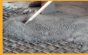
CONCRETE AND REPAIR
