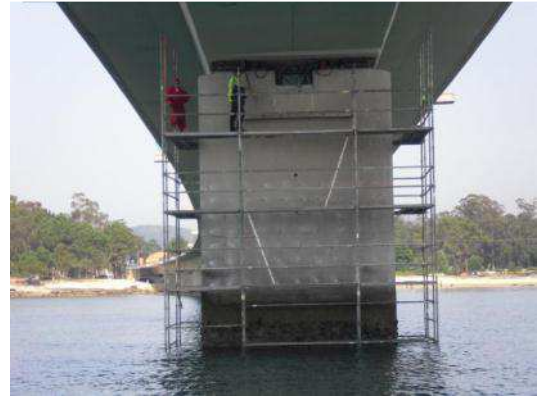
Figure 22: Installation of embedded galvanic anodes
