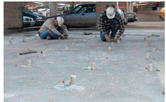
Figure 15: Galvanic anodes linked together for corrosion control in car park deck
