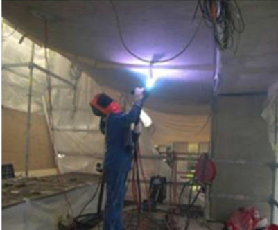
Figure 17: Hot Sprayed zinc coating
