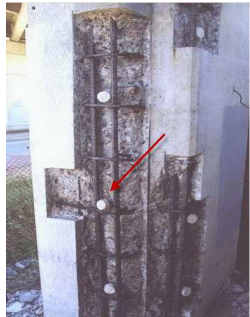
Figure 13: Typical placing for embedded anodes in bridge column patch repair
