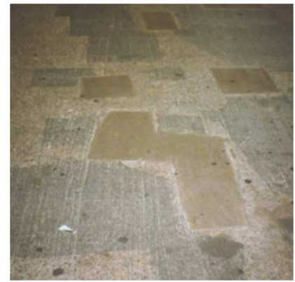
Figure 5: Successive patch repairs due to incipient anode corrosion in car park deck
