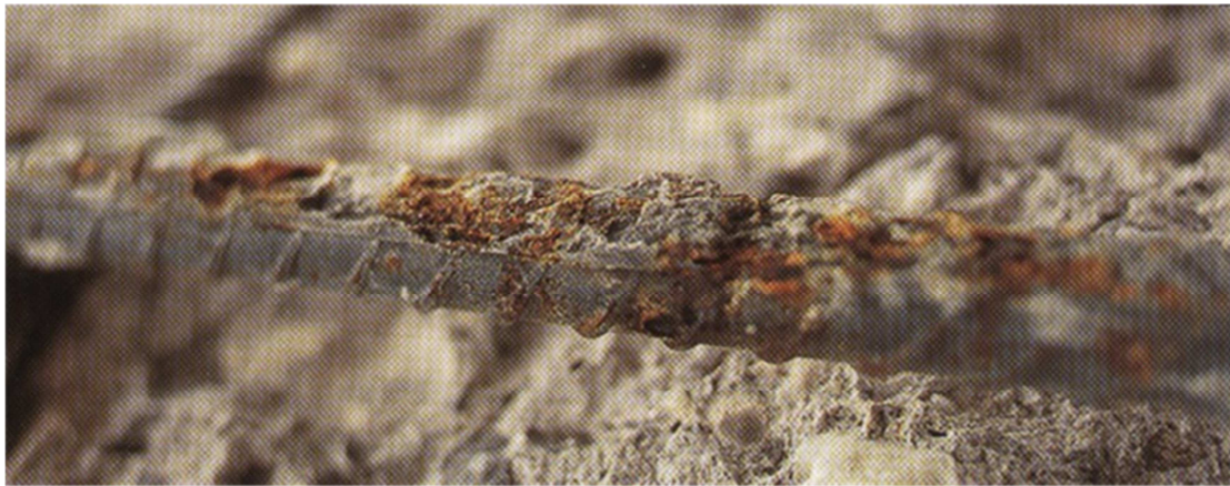
Figure 2: Typical pitting chloride induced corrosion
