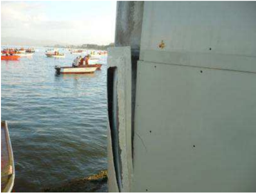
Figure 21: Failed pile jacketing at the Arosa Bridge
