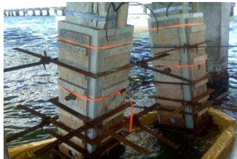
Figure 19: Pile jacketing
