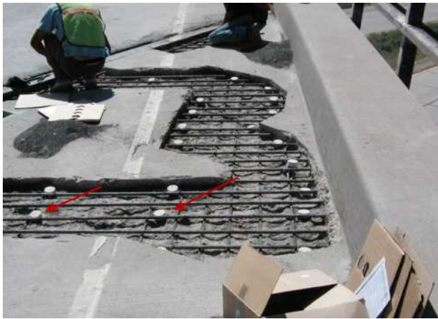
Figure 12: Typical placing with embedded anodes in bridge deck patch repair
