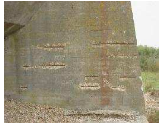
Figure 1: Carbonation induced corrosion with low concrete cover
