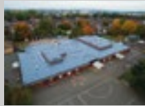
LIQUID APPLIED ROOFING
