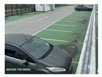
The reinforced concrete multi-storey car park had undergone a major programme of refurbishment to the internal elements of the structure. However, the top deck, split over three levels, had developed splits and cracks, allowing water to enter into the car parking decks underneath.
