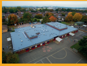
LIQUID APPLIED ROOFING
