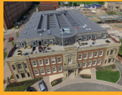
SINGLE PLY ROOFING
