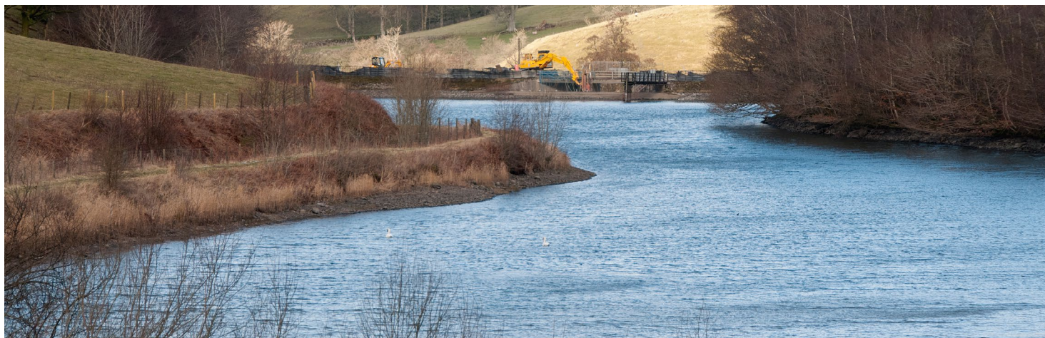
View looking along the reservoir
