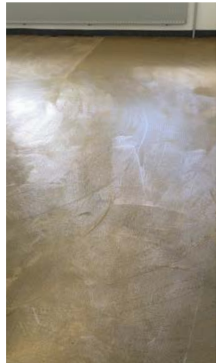
Floor substrate covered with adhesive.
