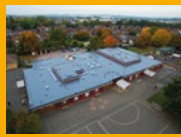
LIQUID APPLIED ROOFING
