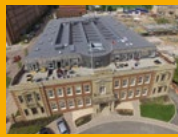
SINGLE PLY ROOFING
