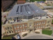
SINGLE PLY ROOFING
