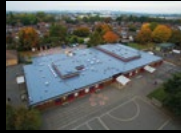
LIQUID APPLIED ROOFING
