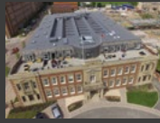
SINGLE PLY ROOFING
