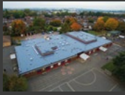
LIQUID APPLIED ROOFING
