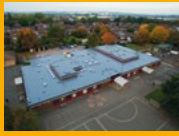
LIQUID APPLIED ROOFING
