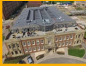
SINGLE PLY ROOFING
