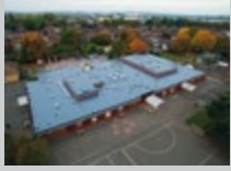
LIQUID APPLIED ROOFING
