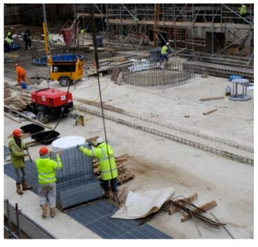
The watertight concrete will effectively form a seal on the Volute channels, which will direct the water into and out of the pumps. A reinforced concrete structure has then been built to support the six individual pumps with six affiliated generators and fuel tanks.
