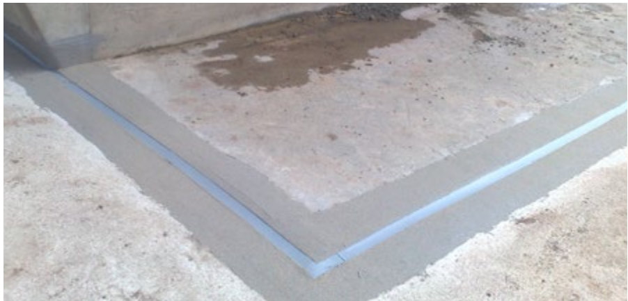
Sealing an expansion joint
