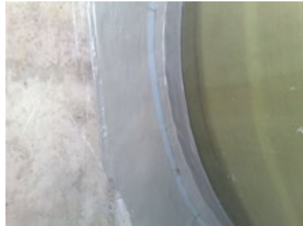
Sealing of a GRP pipe penetration
