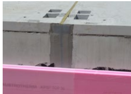
Filling protection of the expansion joint sealing through perimeter insulation
