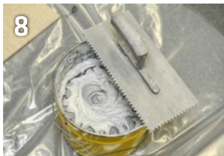
8 Stir for 1 more minute and check that the compound is completely blended. The adhesive is then ready to use and should be applied as soon as possible.
