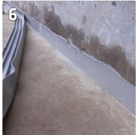
Laying the DFT profile into the adhesive layer
