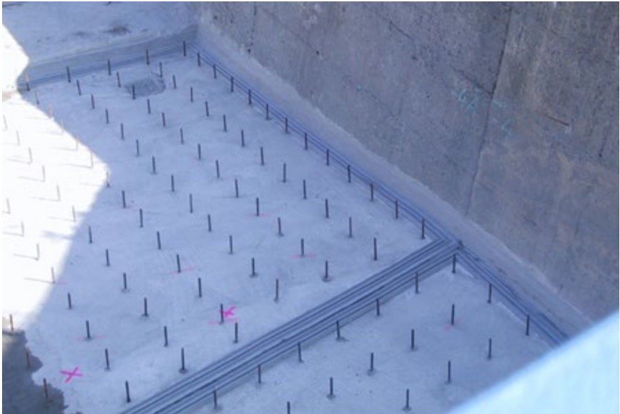
Waterbar profile DFT 330/3 in combination with DFT 330/3KI in the renovation of an existing structure
