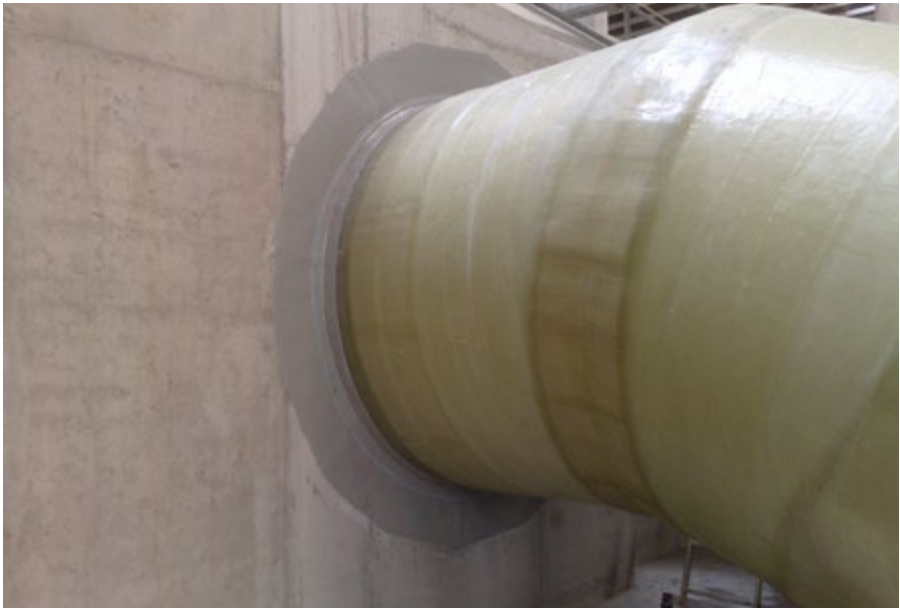
Sealing of pipe penetrations in different dimensions and materials
