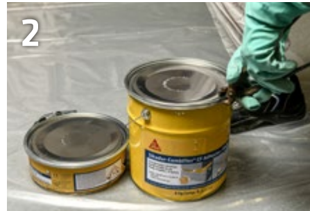
2 Open the container carefully with pliers (use the breakaway line on the snap ring).
