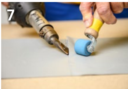
7 Main weld: Next, weld the rest of the overlap area completely. To do this, guide the nozzle of the heat gun so that it slides into the overlap and remains visible 2-3 mm before the leading edge of the seam as the pressure roller follows. In this way, you heat the welding area of the top and bottom and immediately roll the heated areas forcefully with the pressure roller. A welding bead will form along the welded seam.
