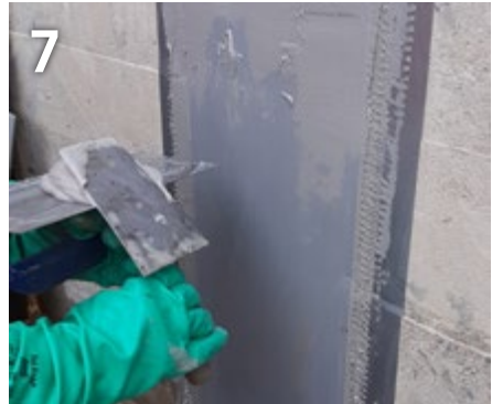
Top layer of the system adhesive in a construction joint
