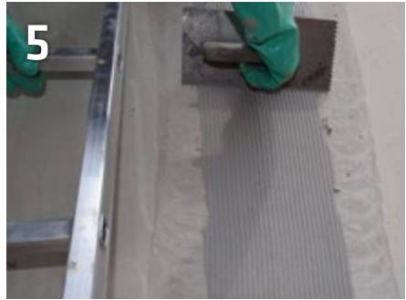
Complete base layer of system adhesive with a 4 mm notched trowel in the area of construction or element wall joints
