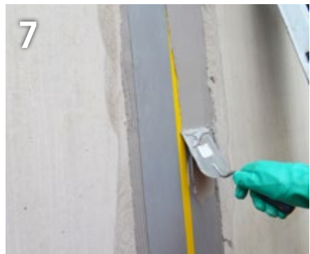
Apply the top layer of the system adhesive when producing expansion joint
