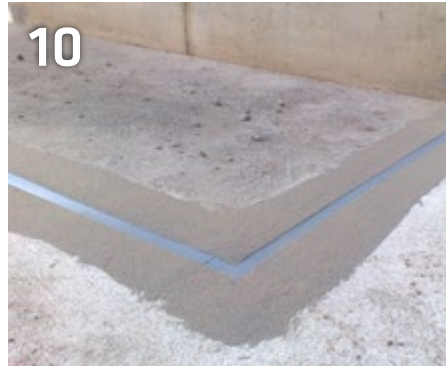
Sanded adhesive layer for subsequent application of coatings
