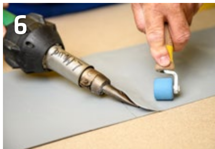
6 Pre-welding: Weld a strip of ca. 10 mm width. Press the heated areas together with pressure roller.
