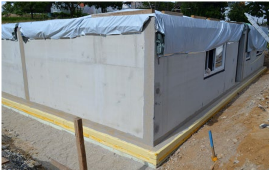
Combination of Sikadur-Combiflex® TF System with the SikaProof® fresh concrete composite system in the concrete slab
