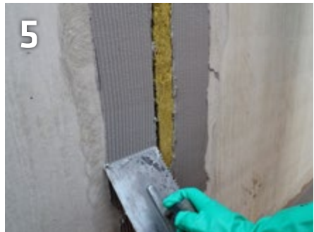
Base layer of system adhesive with 4 mm notched trowel in the case of an expansion joint
