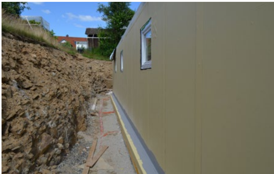
Combination of Sikadur-Combiflex® TF System with the SikaProof® membrane on concrete slab and wall.
