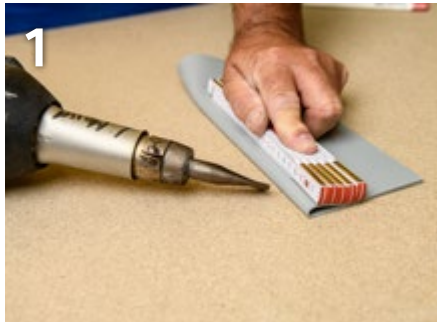
1 Thermoform the jointing tapes lengthwise at an angle.
