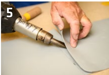
5 Tack the overlap: Spot weld the overlap along the rear edge to prevent it from moving.
