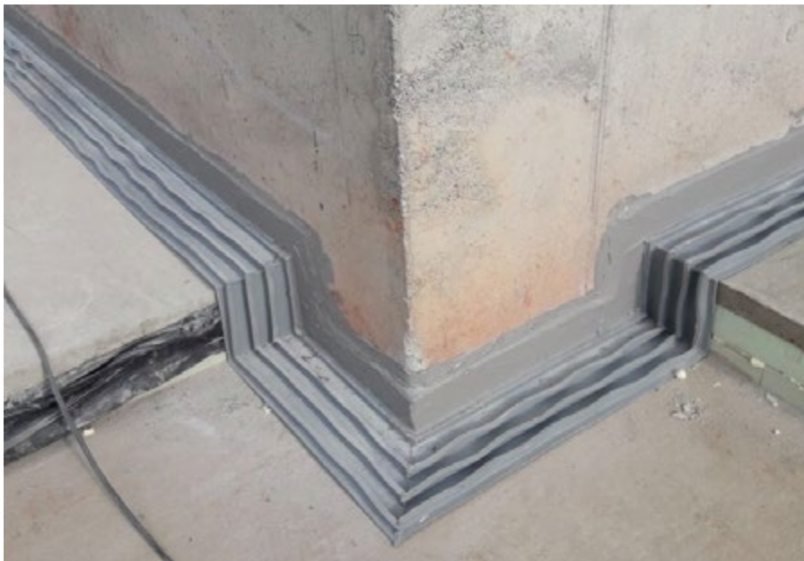
Sealing a connection joint to an existing structure with a profile type DFT 330/3 KI
