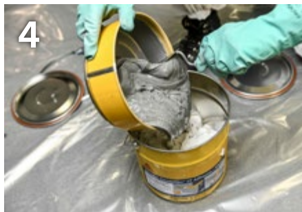
4 Add component B to component A.
