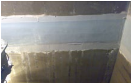
Renovation of a leaking construction joint
