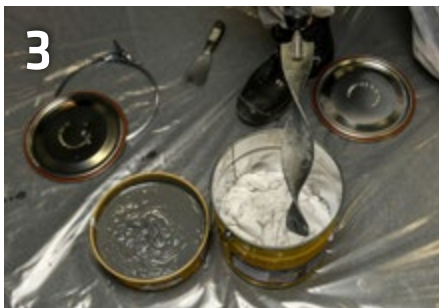
3 Use appropriate mixing paddle to stir in epoxy resin adhesive.
