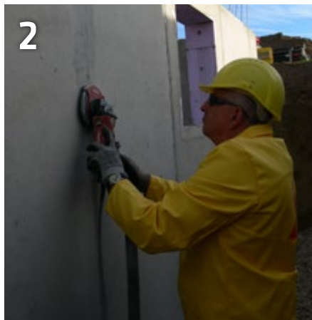
Prepare substrate by grinding with concrete grinding disc
