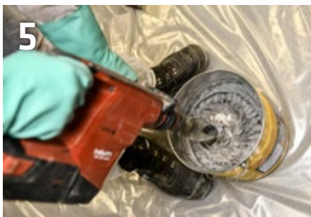
5 Mix system adhesive at low speed for at least 3 minutes (max. 500 rpm.).
