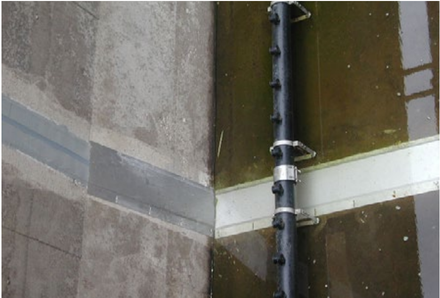
Protection cover with slot construction in a clarifier
