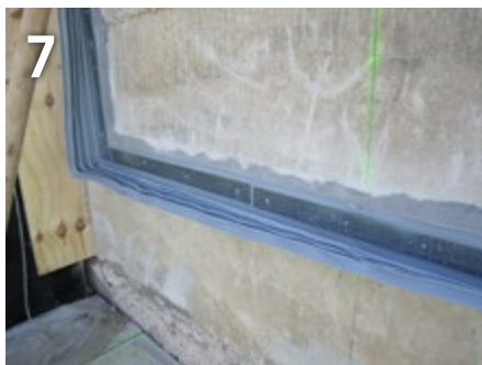
Reinforcing the DFT waterbar profile with a perforated rail
