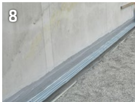
Finished applied DFT waterbar profile
