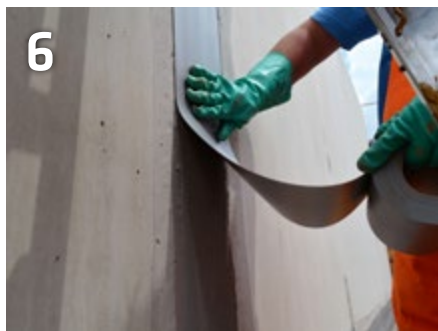
Lay the 1 mm jointing tape into the fresh adhesive layer in the area of a construction joint
