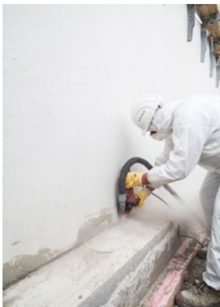
Substrate preparation by grinding the concrete surfaces
