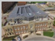
SINGLE PLY ROOFING
