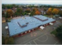
LIQUID APPLIED ROOFING
