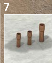
Leaking Penetrations i.e. Pipe Penetrations
