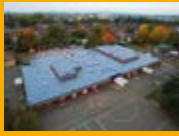
LIQUID APPLIED ROOFING
