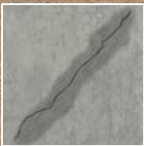
Leaking Cracks
