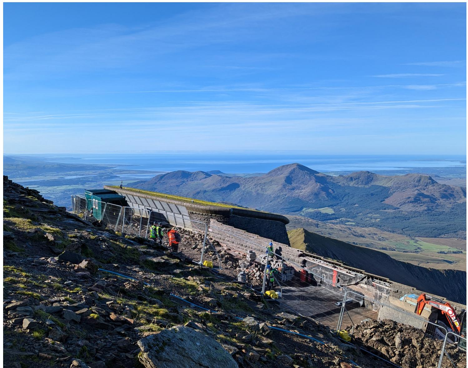
Given the logistical constraints of the visitor centre's remote location, careful management of materials was absolutely imperative. Each day, the project team were required to precisely coordinate which materials were to be brought up and down the mountain. This ensured minimal waste while also adhering to strict weight limits imposed by the railway.
