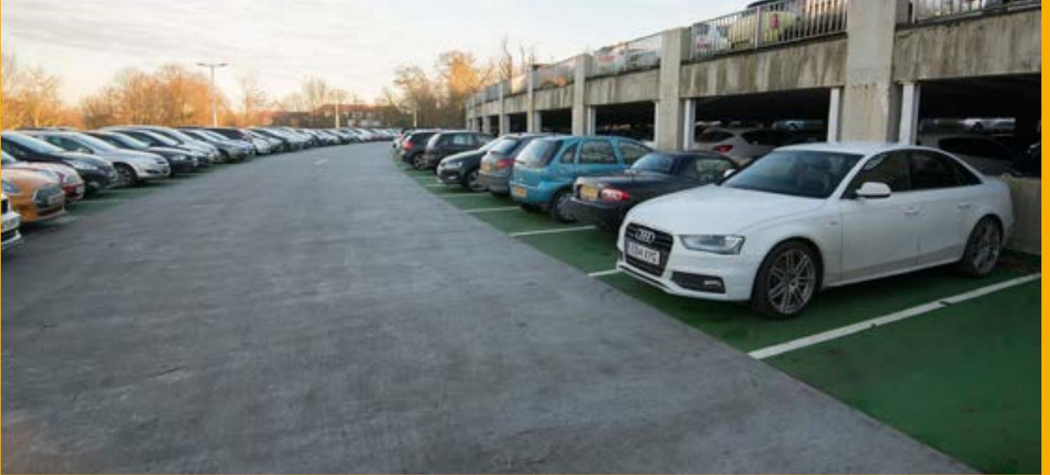
Mastic asphalt was originally used to waterproof both parking decks which have been exposed to the elements since day one. Over time, the surface had badly degraded. Splits in the surface, failed movement joints and blistering were all failures allowing surface water to ingress the structure below resulting in paintwork damage to vehicles parked underneath. The failure of joints combined with cracks in the surface was also creating serious health and safety issues for the car park's users.
