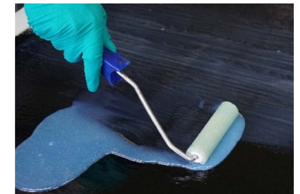
Roller application of SikaBiresin CR169 thix
