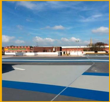
Approximately 4,600m<sup>2</sup> of <u>Sikafloor<sup>®</sup> RB58 Pronto</u> fast-curing decking system was applied to the entire deck area and access ramps to provide a slip resistant and hard wearing waterproof surface. Utilising its fast setting properties, the contractor ensured works could be completed quickly and with minimal disruption to ensure the project remained on schedule.
