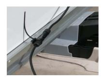
a) The socket of the cable strap for the module cables is clamped into the module frame.
