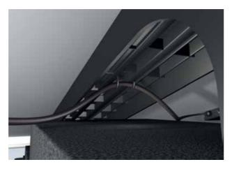
Insert the bundled cables into the mounts in the mounting racks. The cables shall not allowed to swing, and the connectors may not be left on the roof as it may lead to leakage current due to ponding water.
