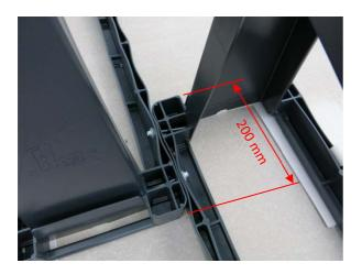
Once the opposite mount ends are aligned in the distance of 0.20 m the mounts are interconnected with two self-drilling screws 6.0 x 75 mm E16.
