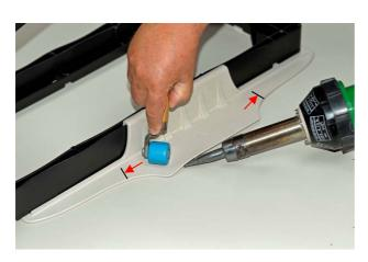
Hand welding of the flaps along the length of 280 mm between the arrow marks on the Sika SolarClick. The same welding process as for the relevant roofing membranes is used.
