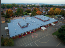
LIQUID APPLIED ROOFING
