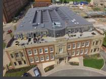
SINGLE PLY ROOFING
