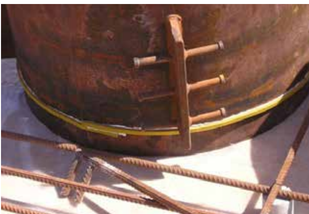
Transitions steel/concrete
