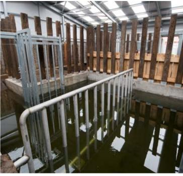
Sika® Watertight Concrete is used in conjunction with the SikaSwell® jointing system, which consists of joint sealing profiles that expand on contact with water, thus ensuring the pool will remain watertight despite the robustness of its occupants.
