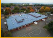
LIQUID APPLIED ROOFING
