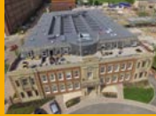
SINGLE PLY ROOFING
