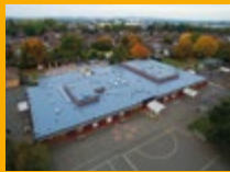
LIQUID APPLIED ROOFING
