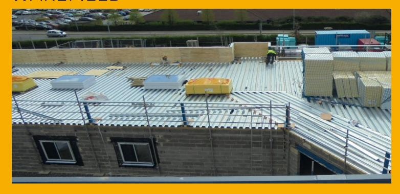
The first phase, which began in January 2017, involved a complex operation to provide a smart, watertight system to an unusually-shaped, multi-directional roof featuring a myriad of details including plant materials and rooflights. For this challenging application, Sika-Trocal® Type 'S' system was selected.
