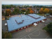
LIQUID APPLIED ROOFING
