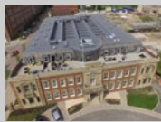
SINGLE PLY ROOFING
