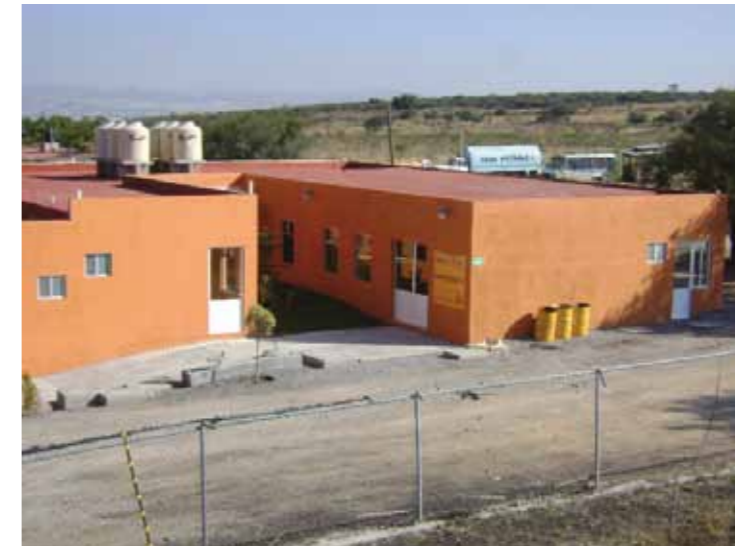
Construction of the boys house
