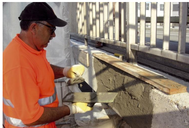
Figure 9: Hand application of repair mortar Sika MonoTop®-4012.
