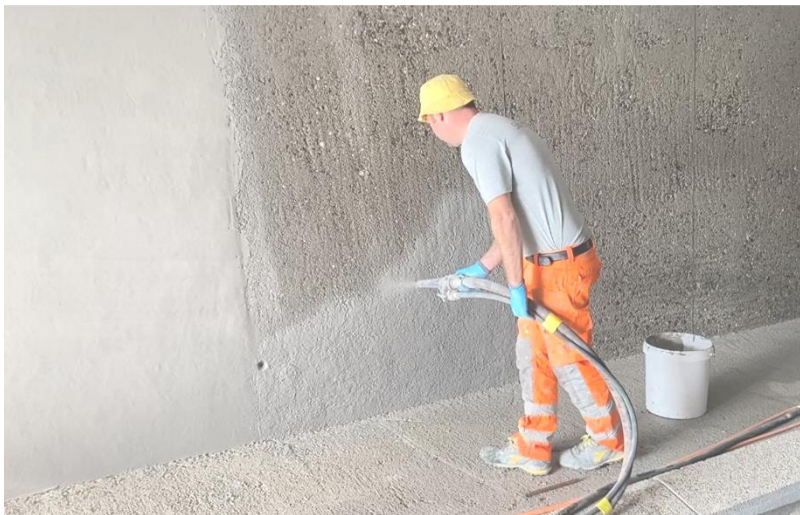
Figure 11: Application of Sika MonoTop®-3020 by spray and hand application.
