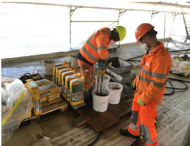
Figure 3: Mixing and pouring into the pump for pumping.
