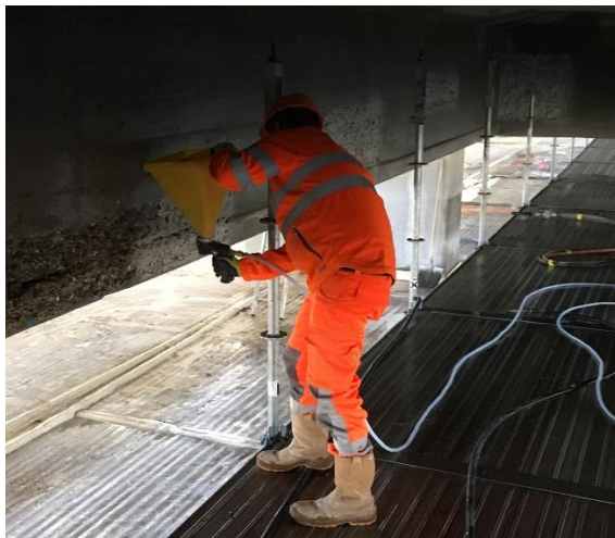
Figure 6: Application of bonding primer Sika MonoTop®-1010 with Hopper gun.
