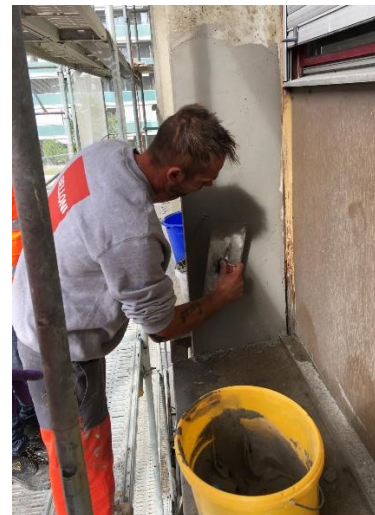
Figure 11: Application of Sika MonoTop®-3020 by spray and hand application.
