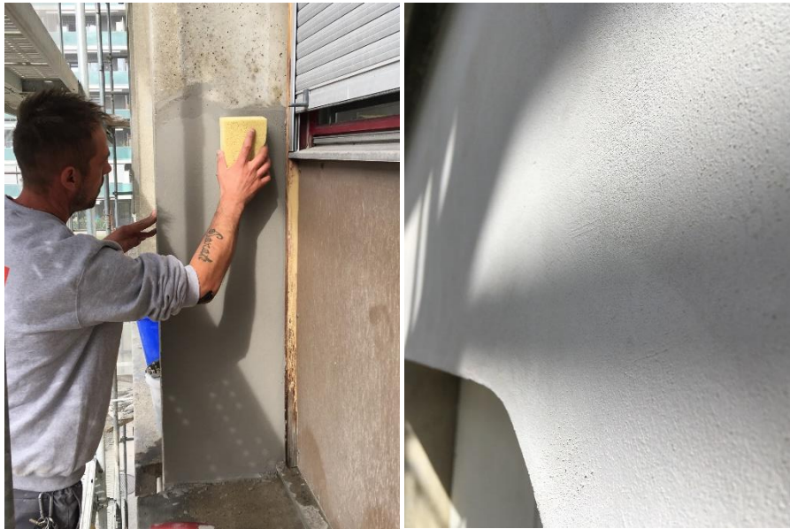
Figure 12: Finishing the levelling mortar Sika MonoTop®-3020 with a sponge.
