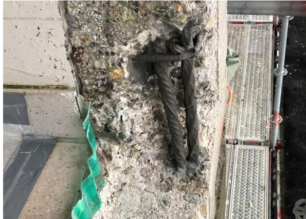
Figure 5: Applied corrosion protection SikaTop® Armatec®-110 EpoCem® on steel rebars.
