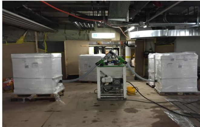
Figure 4: Inotec mixing pump with dust free material supply in one-way containers (OWC).
