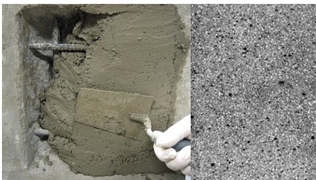
Figure 7: Hand applied mortar.
