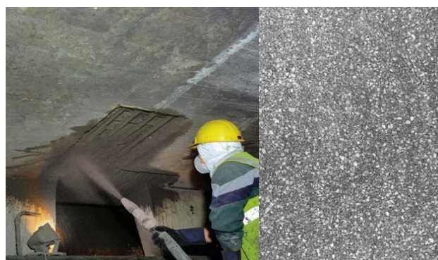
Figure 8: Machine applied mortar - more densely packed.
