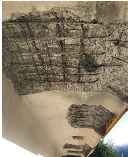
Figure 1: Substrate preparation by concrete removal with high water pressure and placing of formwork (shown on the right side of the photo).
