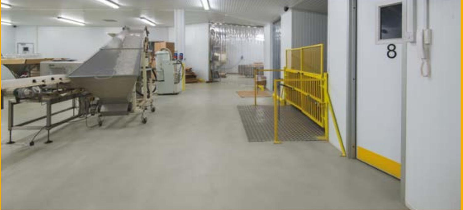
Highly resistant to chemicals, fatty acids and temperature, Sikafloor®-20N PurCem® is a polyurethane modified cement screed offering excellent strength and because it normally requires no primer, its installation is considerably less complex than many other systems.
