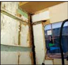
Don't ignore the smell of damp and mould
