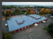
LIQUID APPLIED ROOFING
