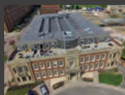
SINGLE PLY ROOFING
