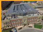
SINGLE PLY ROOFING
