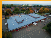
LIQUID APPLIED ROOFING
